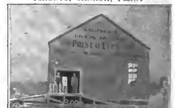
SAN FRANCISCO CHARGING PLANT
